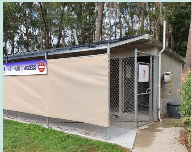
Widened paths, new roofing and weather barrier in the pound.
